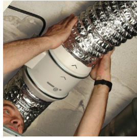
Connect the ducts.
