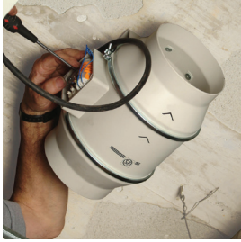
Carry out the wiring connections.
