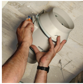
Place the impeller and motor.
