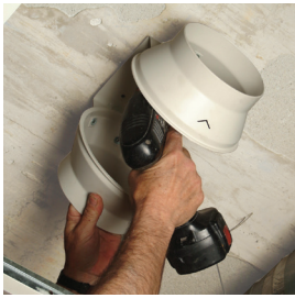
Fix the support bracket.
