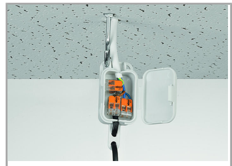
Pendant light connection in suspended ceilings
