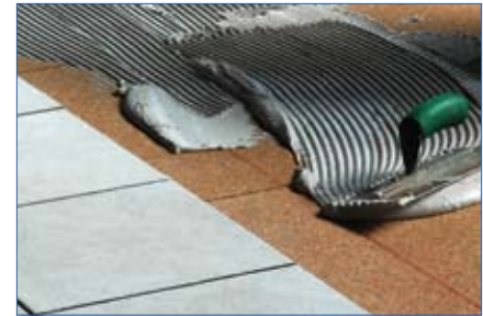
A direct bonded Ceramic Tile installation over AcoustiCORK, as per NTCA Handbook Method # F135-07.
